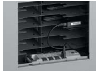
Has a 120-V receptacle for each device.
