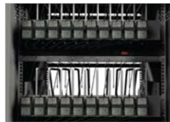
Power brick lacing stores power bricks easily and neatly (medium- and large-shelf models only).
